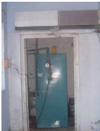
Figure - 10: Absorption-Type chiller of 3 tons capacity
