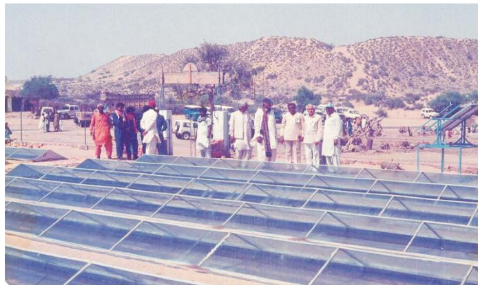
Figure - 2: Solar Water-Desalination Plant, Vajuto-District Tharparkar
