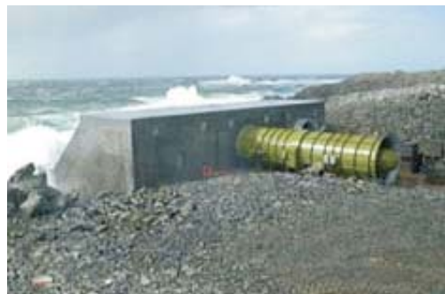
Figure - 13: The World's First Commercial Wave-Power Station, on the Scottish Island of Islay
