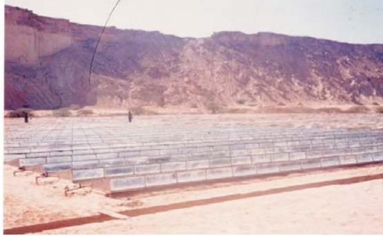
Figure-3: Solar Water-Desalination Plant, Gwader
